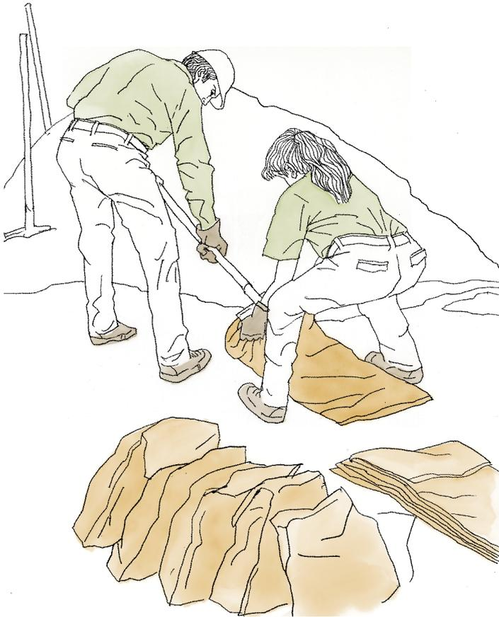
Figure 1: Proper sandbag filling
