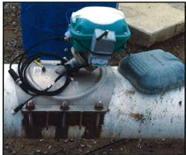
Wildeye units monitoring a Seametrics AG 2000 (left) and a McCrometer McMag 3000 (right)
