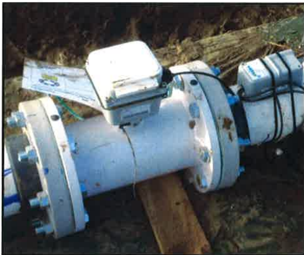
Wildeye units monitoring a Seametrics AG 2000 (left) and a McCrometer McMag 3000 (right)
